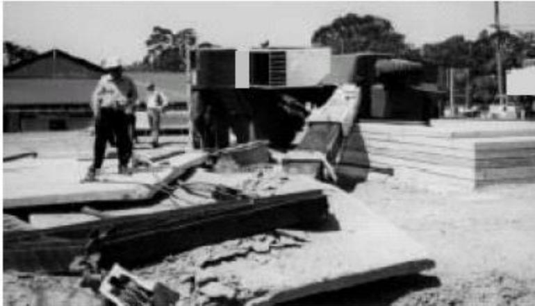
*Diagram 7 – Rubber tyred pick and carry crane overturned*
