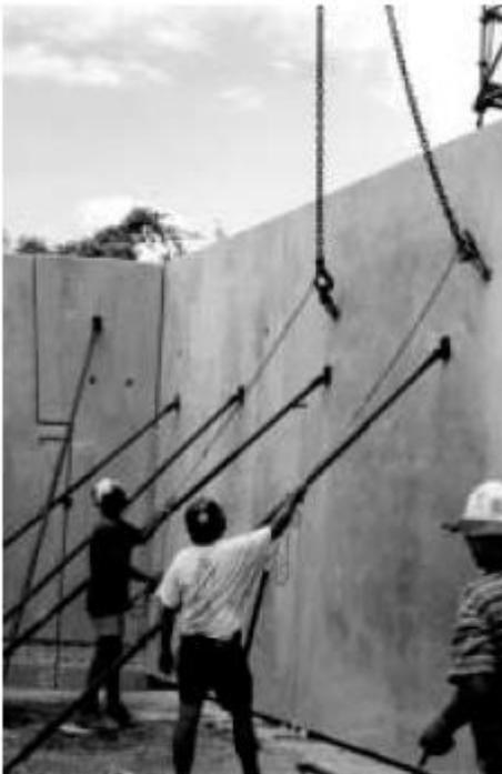
*Diagram 9 – Lifting clutch release lines*
